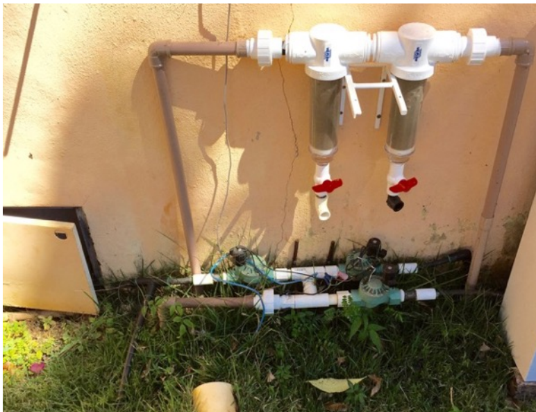
Photo 2: Irrigation water filters (200 Mesh)
